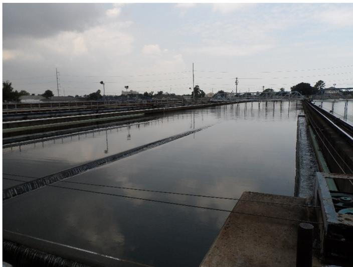
**Figure 3-9: L Basin Sedimentation Basin**
