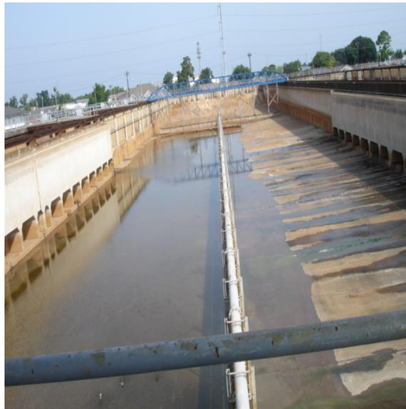
**Figure 5-2: Dewatered Sedimentation Basin with Ground Water Infiltration**
