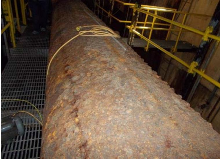
**Figure 3-12: Deteriorated Condition of Raw Water Piping Filter Nos. 1-10 at Sycamore**
