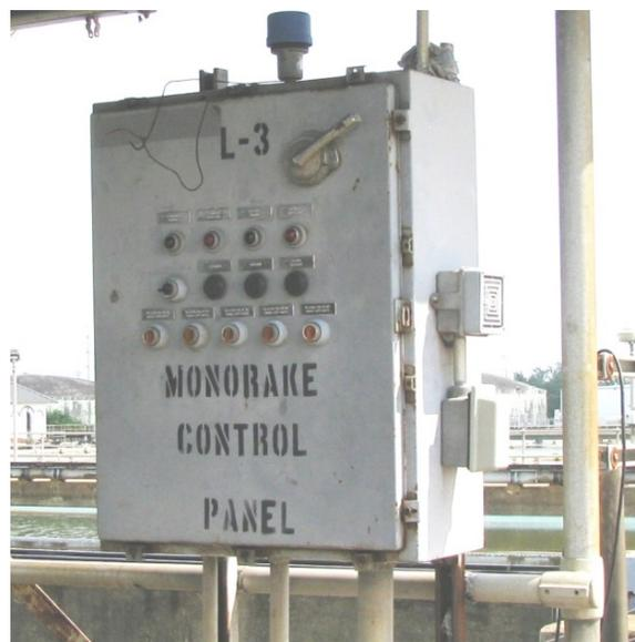
**Figure 4-2: L3 Basin Control Panel**
