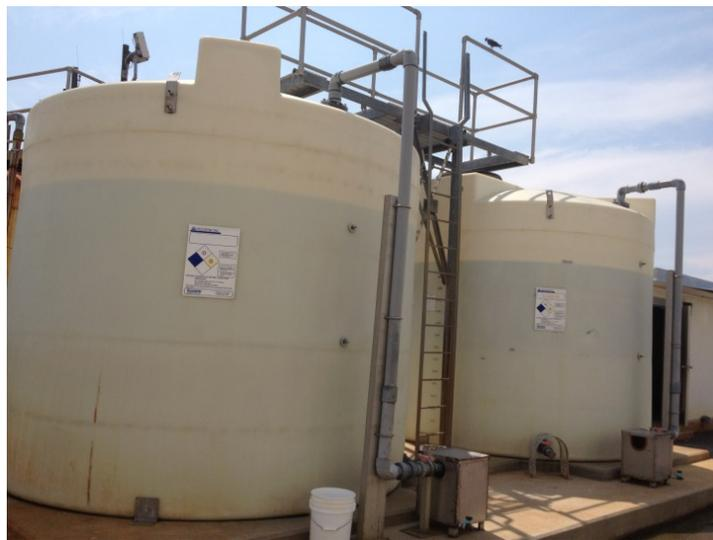
**Figure 3-57: Polymer Storage Tanks**
