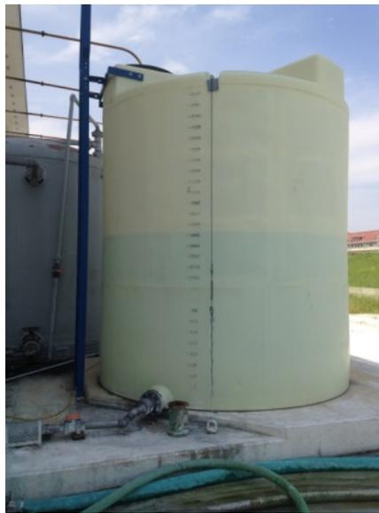
Figure 3-54: Polyphosphate Storage Tank
