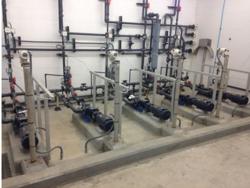
**Figure 3-29: NaOCl Feed Pumps**
