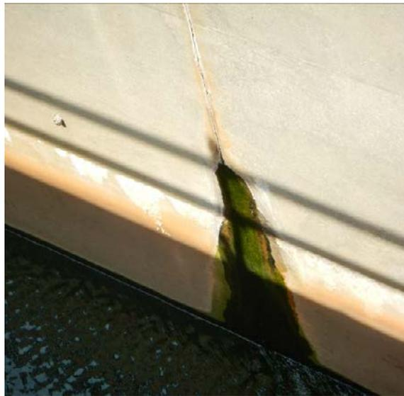
**Figure 5-9: Water leak from a vertical construction joint at the Claiborne Filter Gallery**
