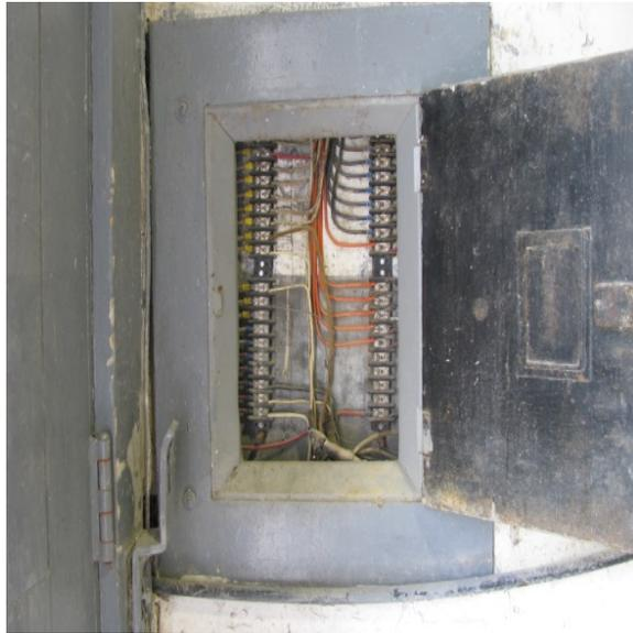
**Figure 4-5: Deteriorated Junction Box**
