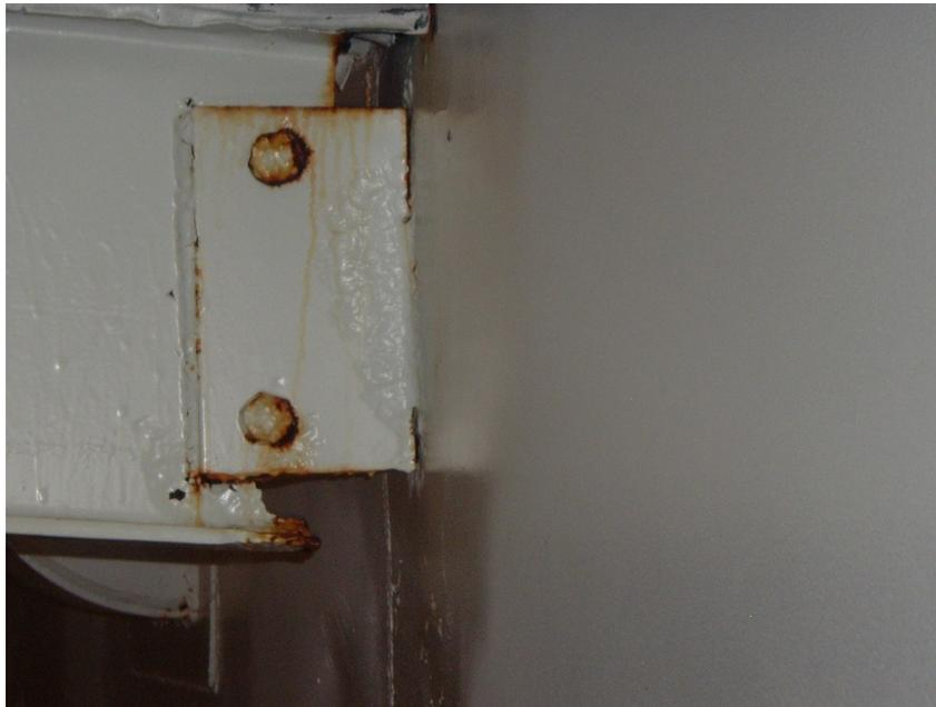
**Figure 5-12: Corrosion of GST Roof Beams**
