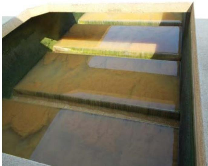
**Figure 3-13: Example of Debris in Filter**
