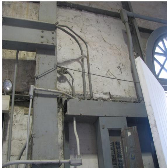
**Figure 4-4: Deteriorated Electrical Equipment**
