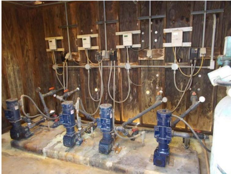
**Figure 3-43: Ferric Sulfate Feed Pumps**
