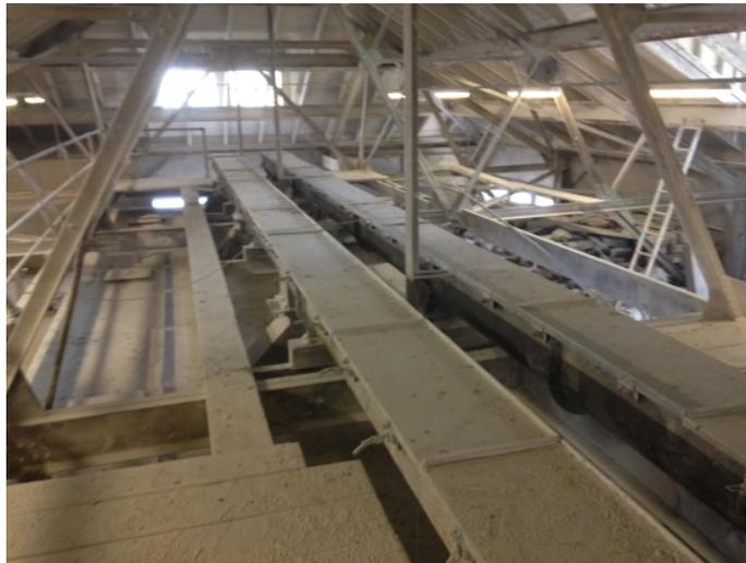
**Figure 3-34: Chemical Building Attic Showing Horizontal Lime Conveyors**
