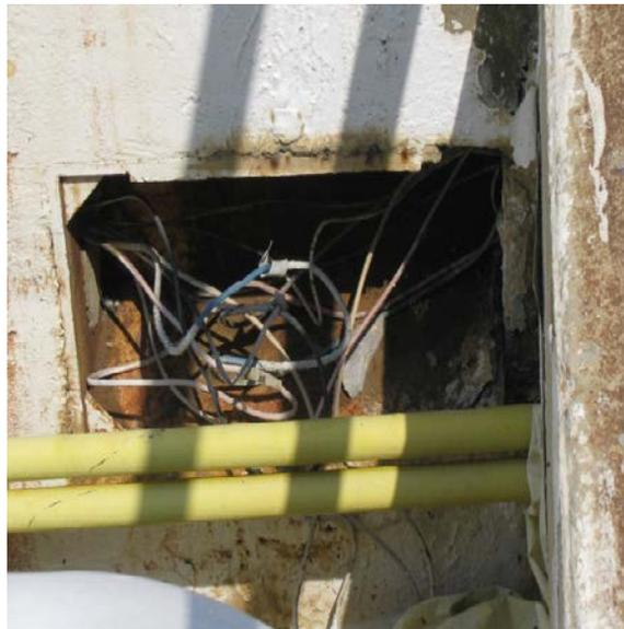
**Figure 4-3: Junction Box with Deteriorated Wiring and Missing Cover**
